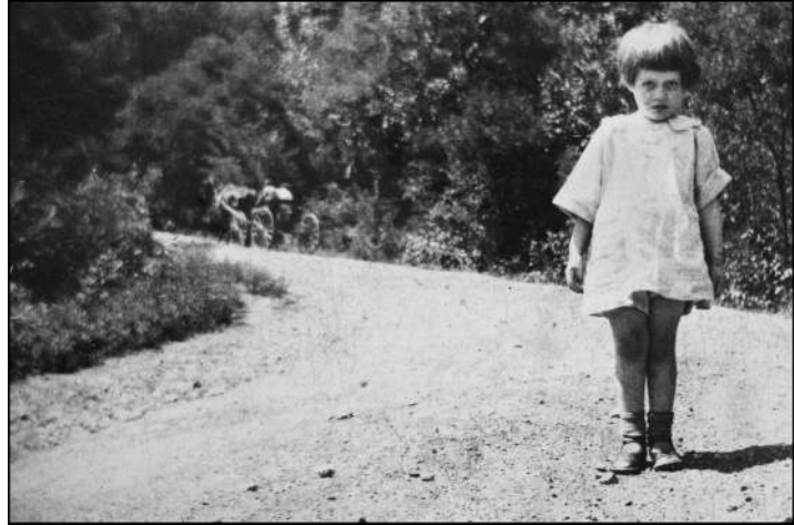
Bunny Hammer Market Street Hill Rd c. 1927
